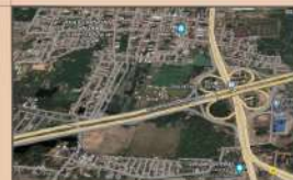
JUST 2 MINS 400 FT ELEVATED HIGHWAY - NH48
